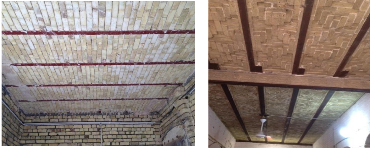
Figure (1): Traditionally jack arch slab in south of Iraq
