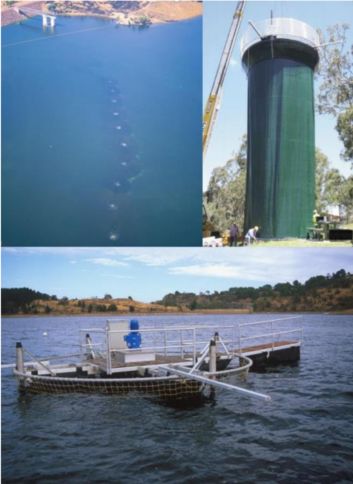
Figure 8: Destratification systems. Clockwise from top left: 10 bubble plumes, draft-tube mixer and unconfined mixers (Sherman et al., 2010)
