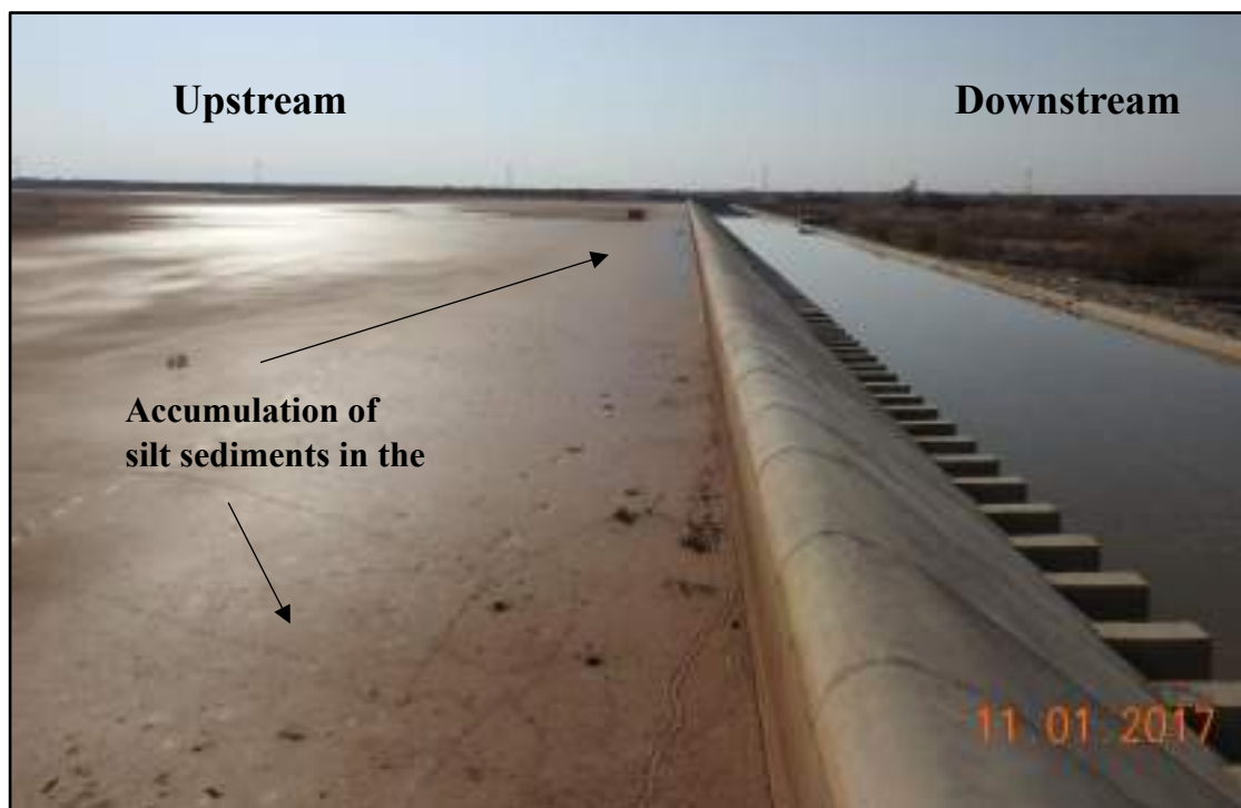
Fig. 5.11 Siltation problem in dam reservoir (Al-Sudani, 2018)
