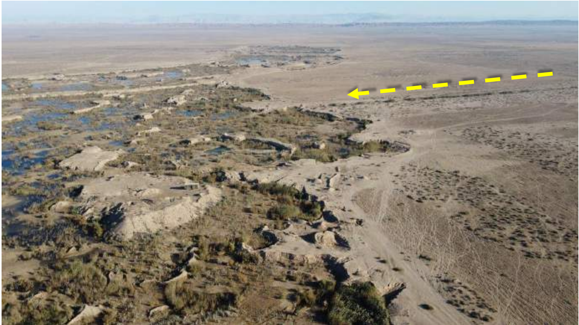
Fig. 5.26 Influence of quarries activity on the canal project
