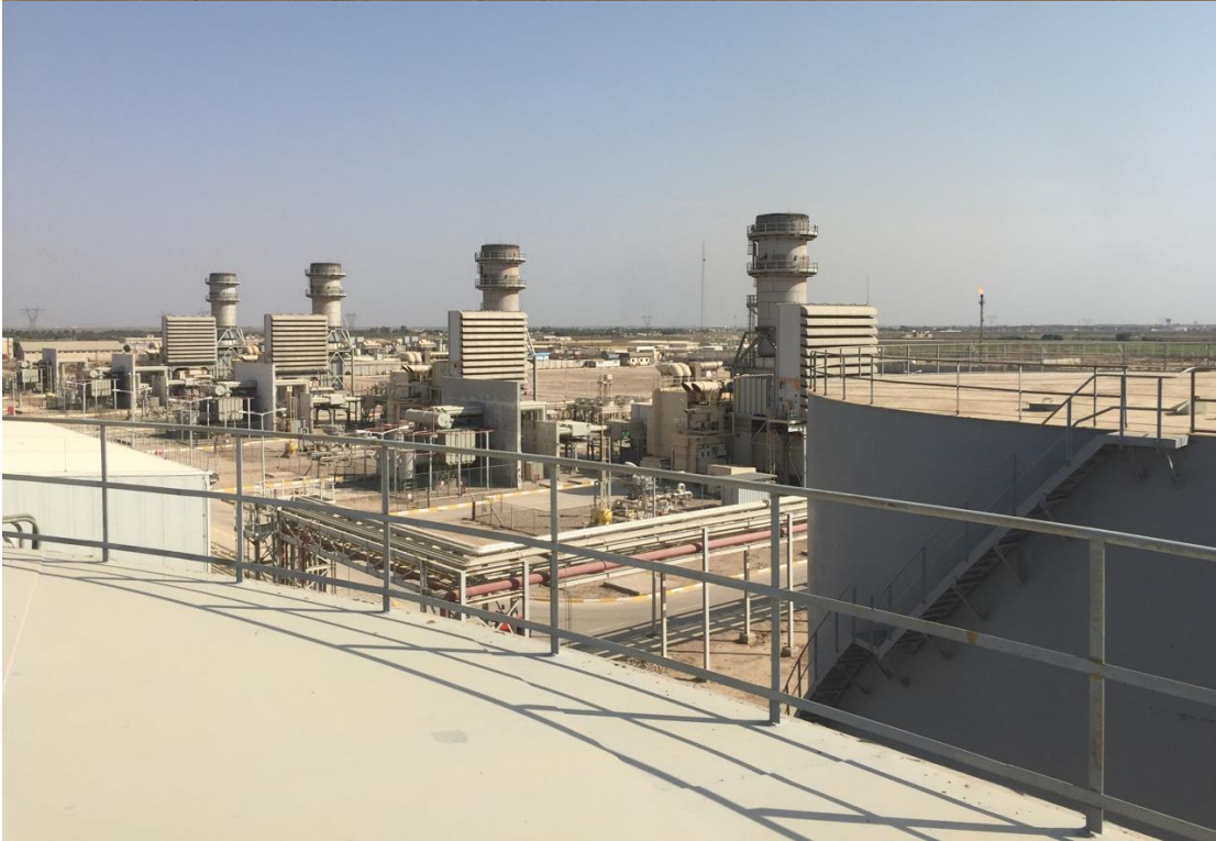
Figure 6.1: Amara Gas Turbine Power Plant
