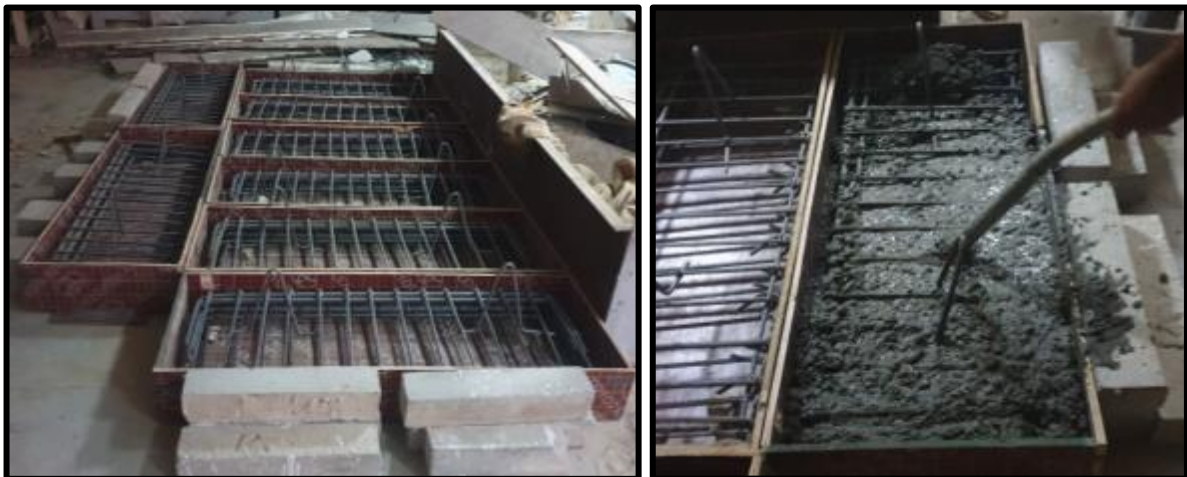
Fig. 4: Steel Reinforcement of deep beams.
