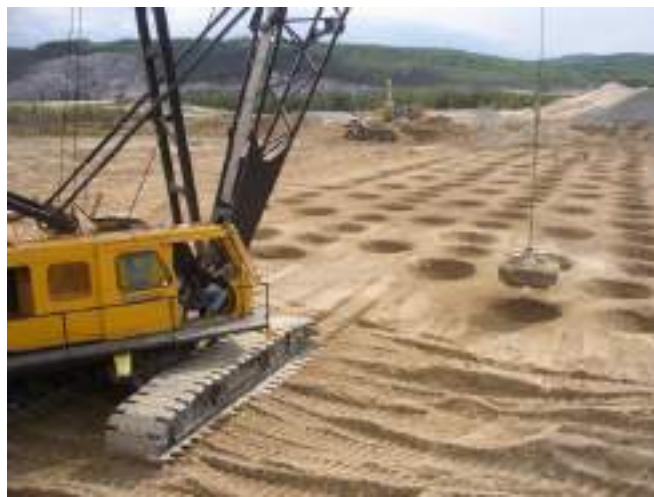
Figure 2-1 Shallow stabilization (dynamic compaction)
