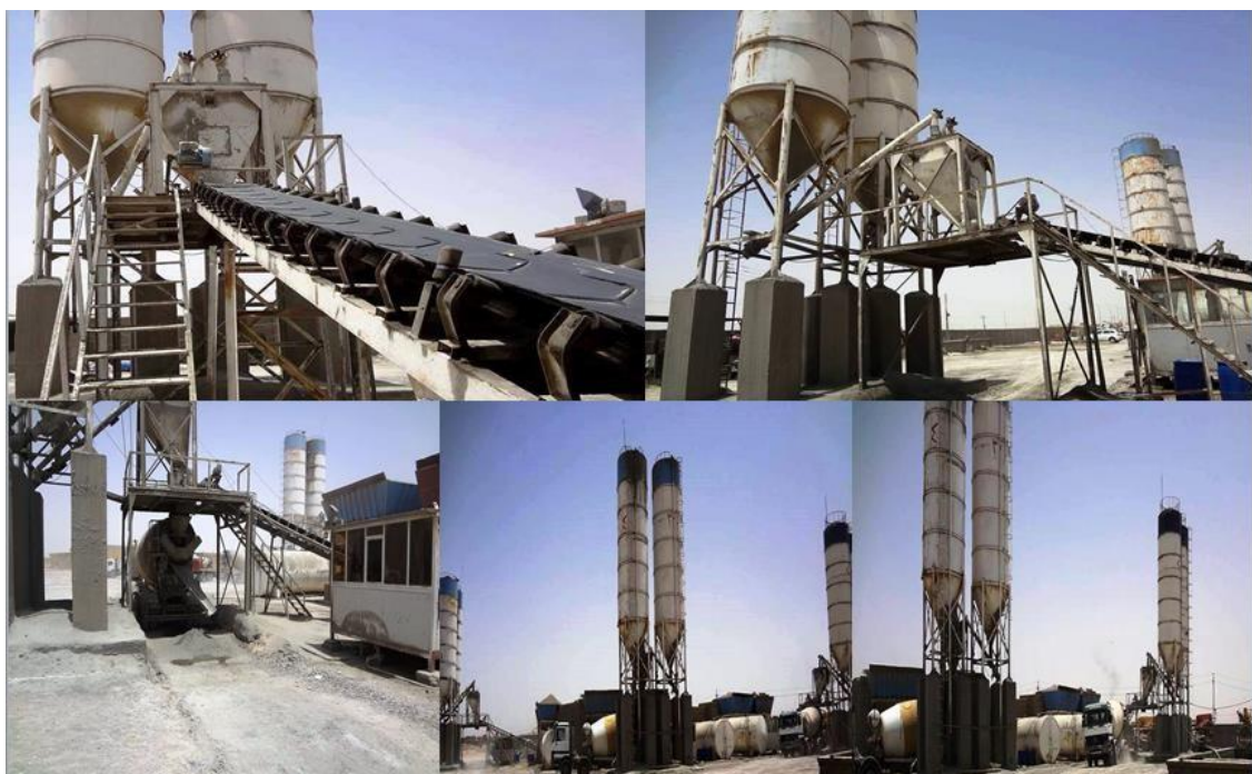
Fig. 7. AL-Senaf Ready Mix Concrete batching plant ( Researcher ).
