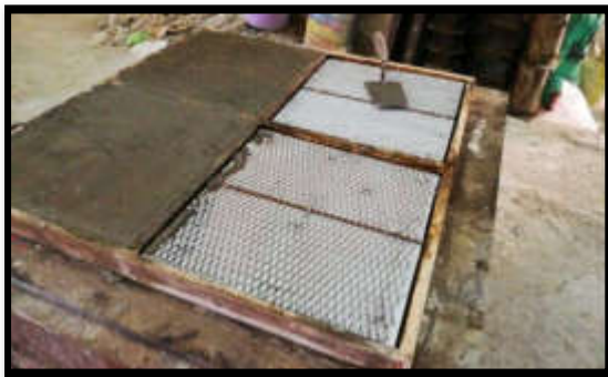
(c) Casting of the top skin ferrocement layer.
