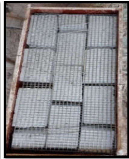
(c) Apply reinforcement cage for top layer.
