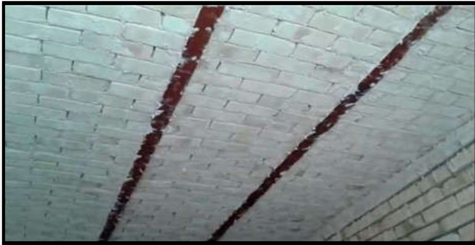
Figure. 1-1: Jack arch slab after construction.
