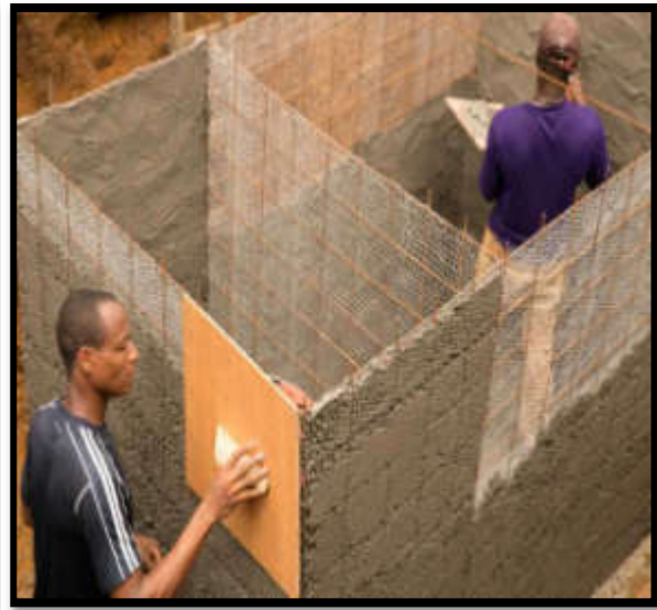
(b) Construction septic tank [13].
