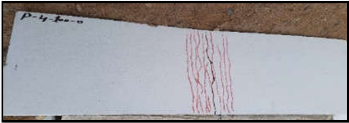
(e) Mode of failure for P-4-100-0 specimen.
