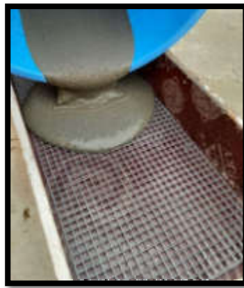
(b) Apply cement mortar.
