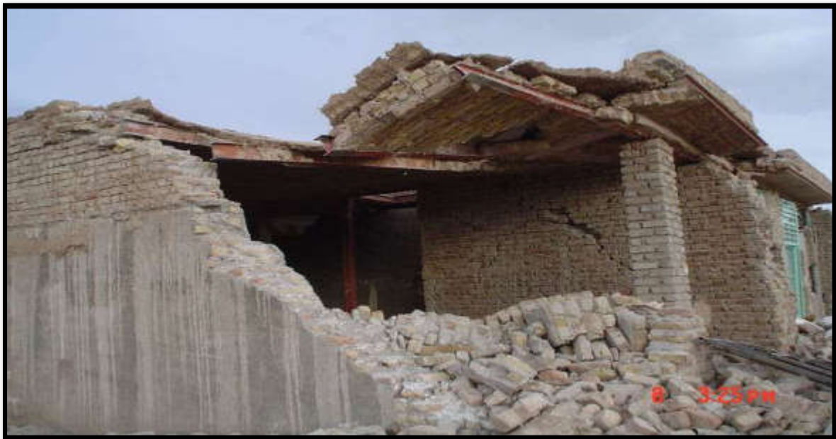
Figure. 2-2: Failure modes of masonry structures [8].
