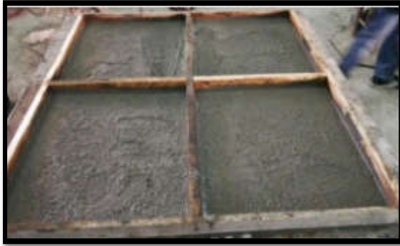
(a) Casting of the bottom skin ferrocement layer.
