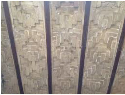
(a) A historic house's jack arch slab, about 1830.
