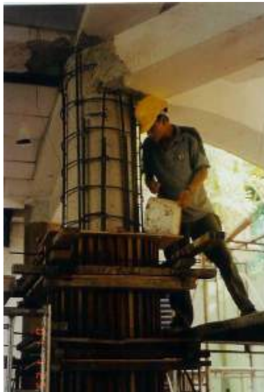
Plate (1.2) Size enlargement of concrete columns.
