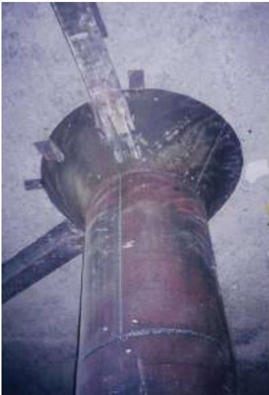
Plate (1.1) Strengthened concrete column with steel plate.
